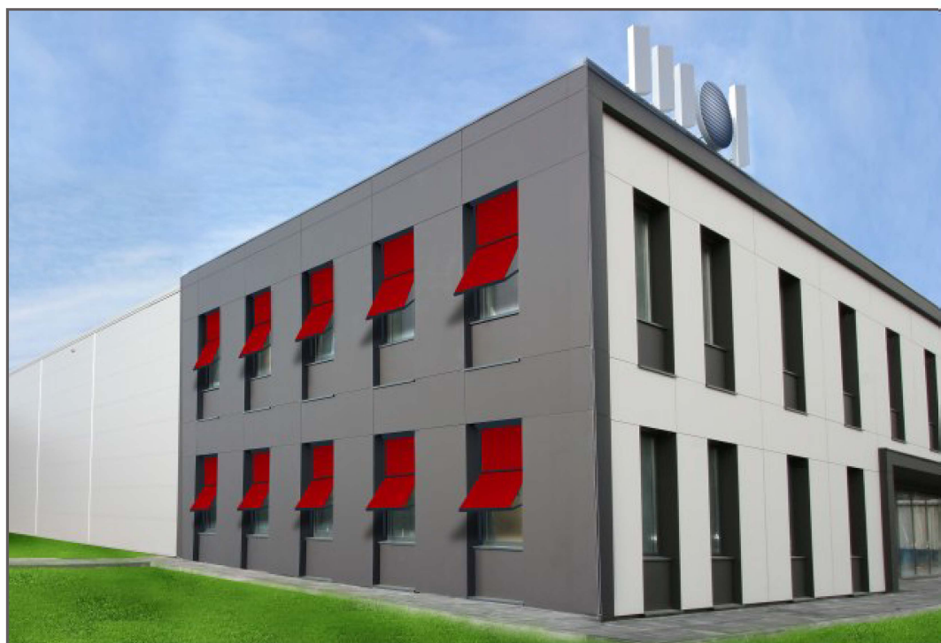
MOL office building
